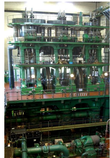
Kempton's 1000 ton triple expansion steam pumping engine
