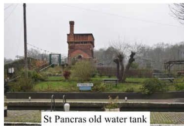
St Pancras old water tank
