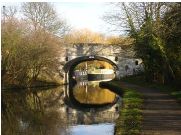
Bridge on Grand Union Canal
